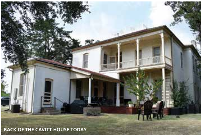
BACK OF THE CAVITT HOUSE TODAY
